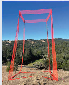
Cell phone tower poles at San Domenico where Verizon has committed to installation this year thanks to tremendous community support and SHHA advocacy.
